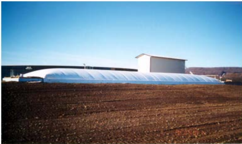
Figure 2-6 A dairy farm anaerobic digestion system
